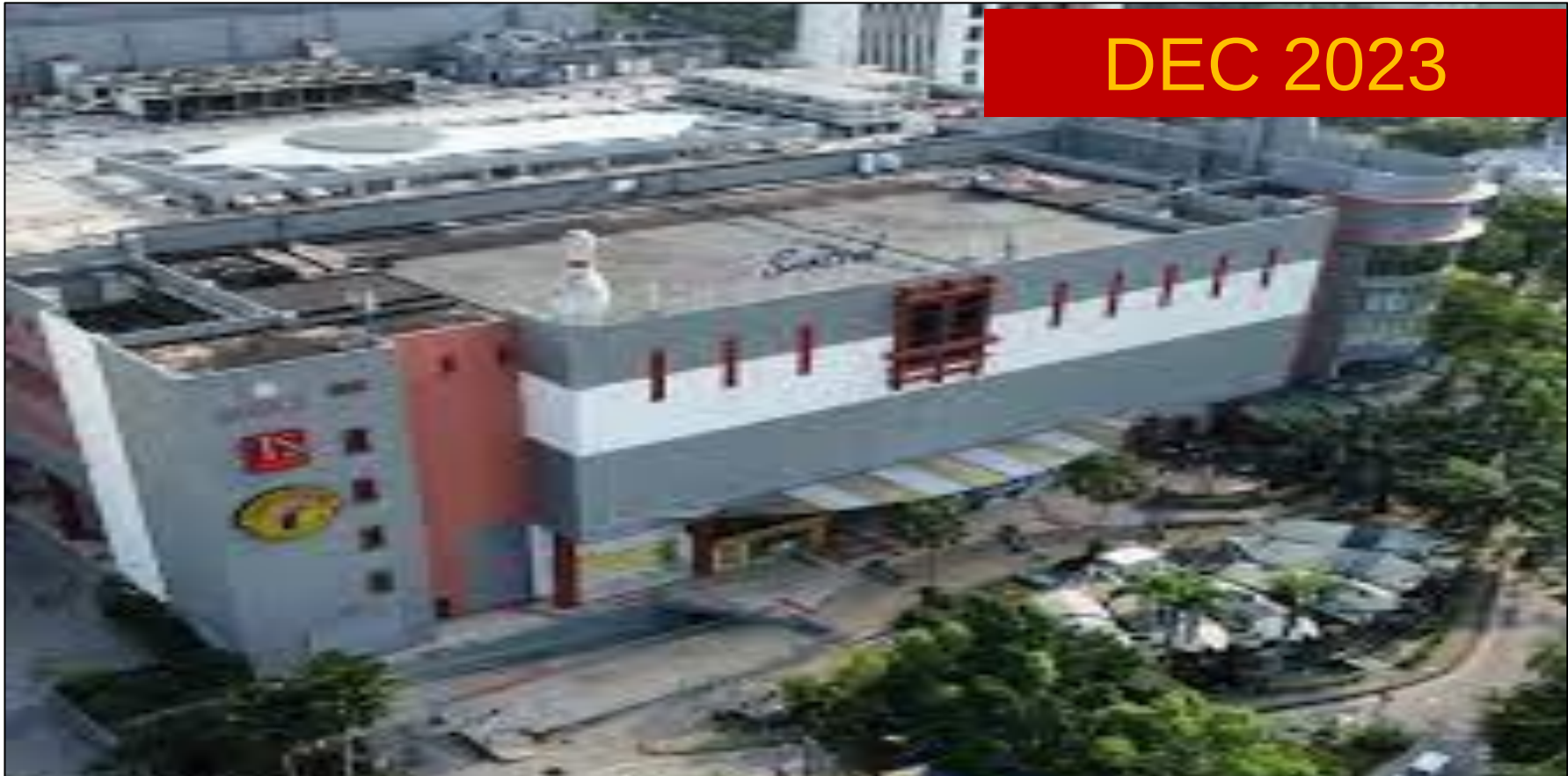
RM178 million (RM406 psf) Plaza Alam Sentral Mall, Shah Alam NLA: 438,930 sf
