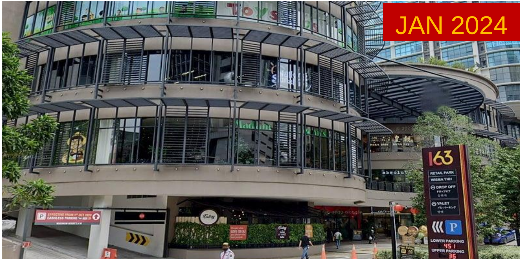
RM215 million (RM841 psf) 163 Retail Park, Mont Kiara NLA: 255,535 sf est.
